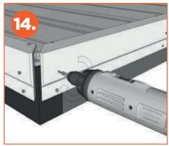
Measure the required amount of Edging trim and cut down to size, mitre down the ends at 45° angles if installing around corners (fig. 13) Cover the deck edge with corner trim and attach with screws
